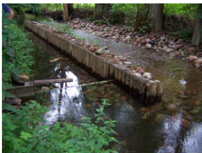
(3) The bypass on the Lake Roofensee weir allows biological permeability for aquatic organisms
