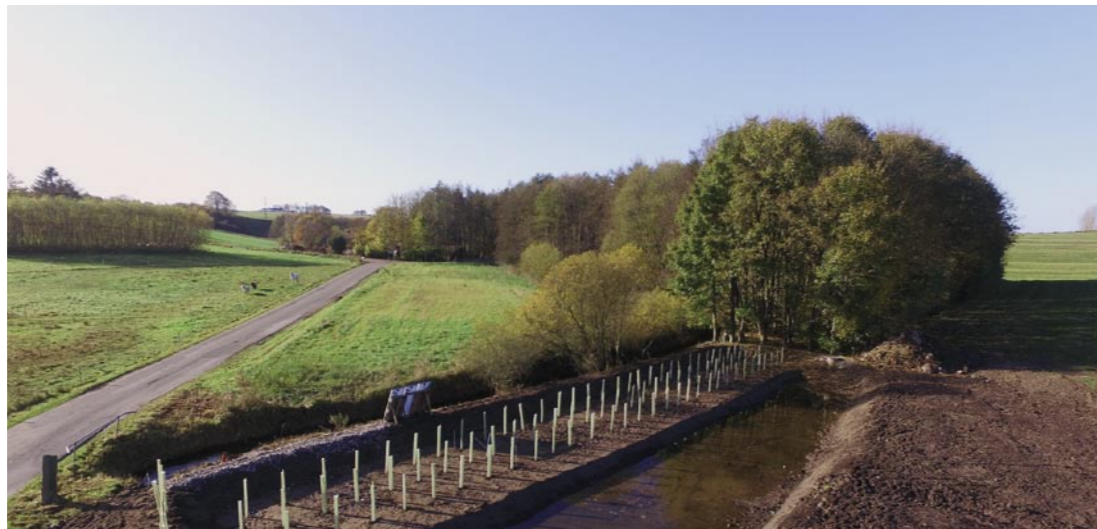
Trees within the infiltration zone optimize the infiltration capacity of the buffer area.
